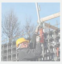
Safety on the opposite side of the formwork is provided by a guardrail consisting of three system components and guardrail boards: the brace connector with a supplementary guardrail post holder is mounted on the panel; the guardrail posts can then be simply inserted.
