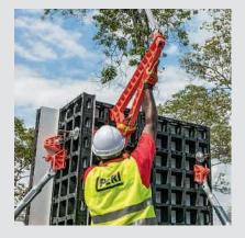
Firstly, the post is inserted into the scaffold bracket, then the bracket is simply hooked into the panel. Subsequently, 5 cm thick scaffold boards and guardrail boards are installed and fixed in position with screws or nails.
